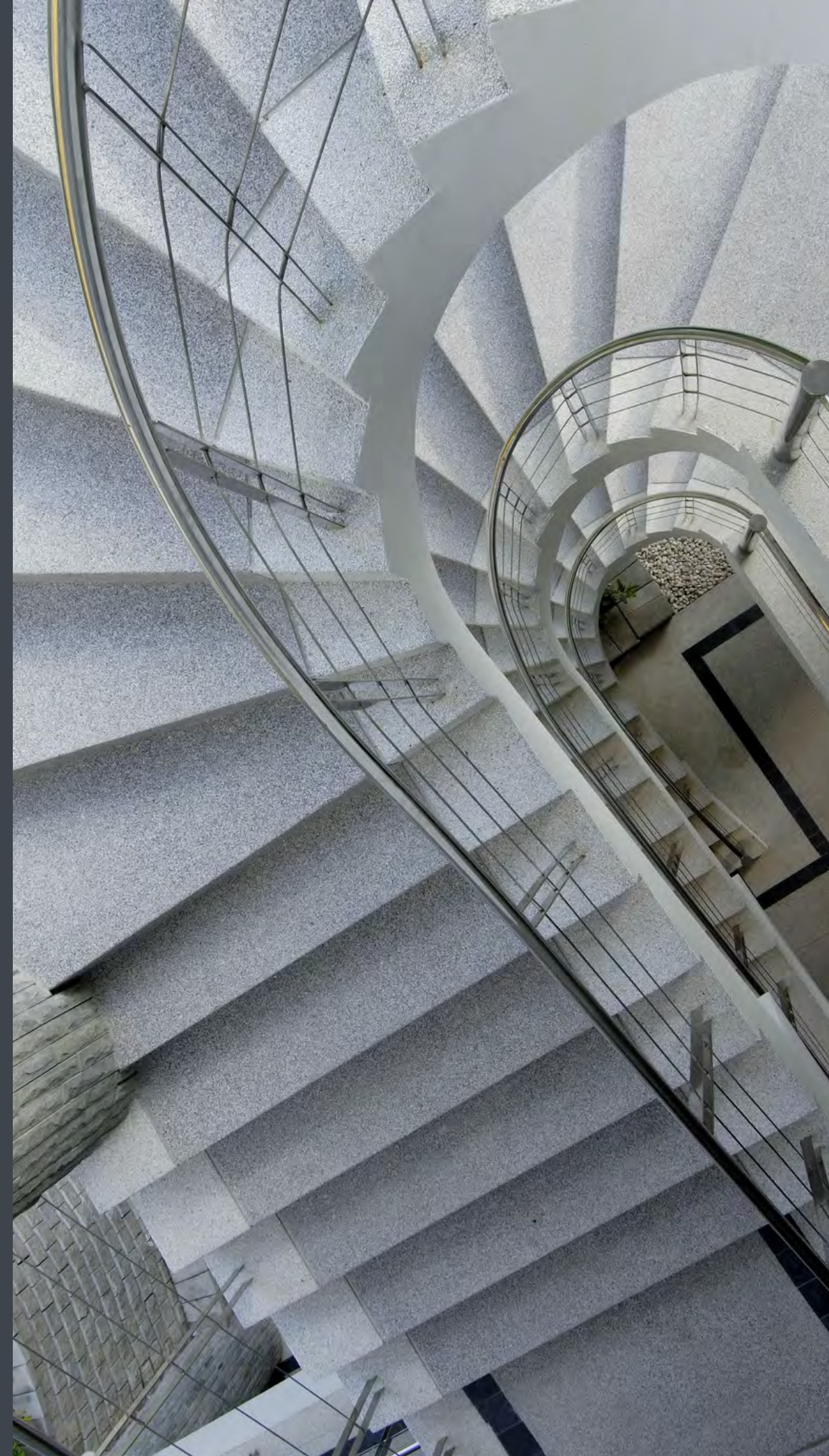
Spiral Staircase - Accenta Project 2006
